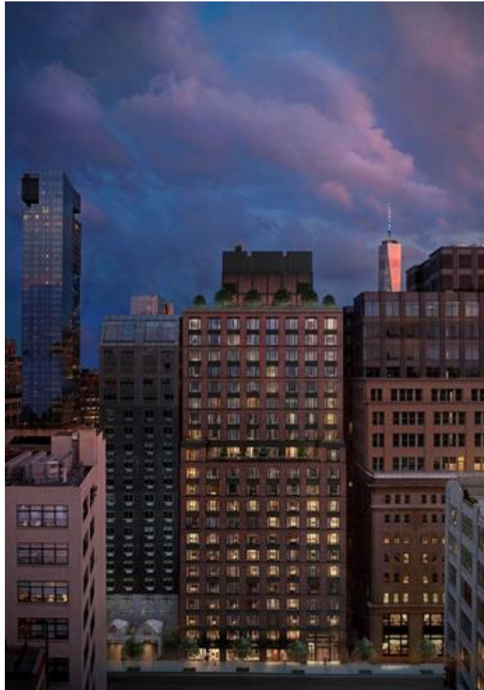
The 70 Charlton development has two 22-story connected towers.
