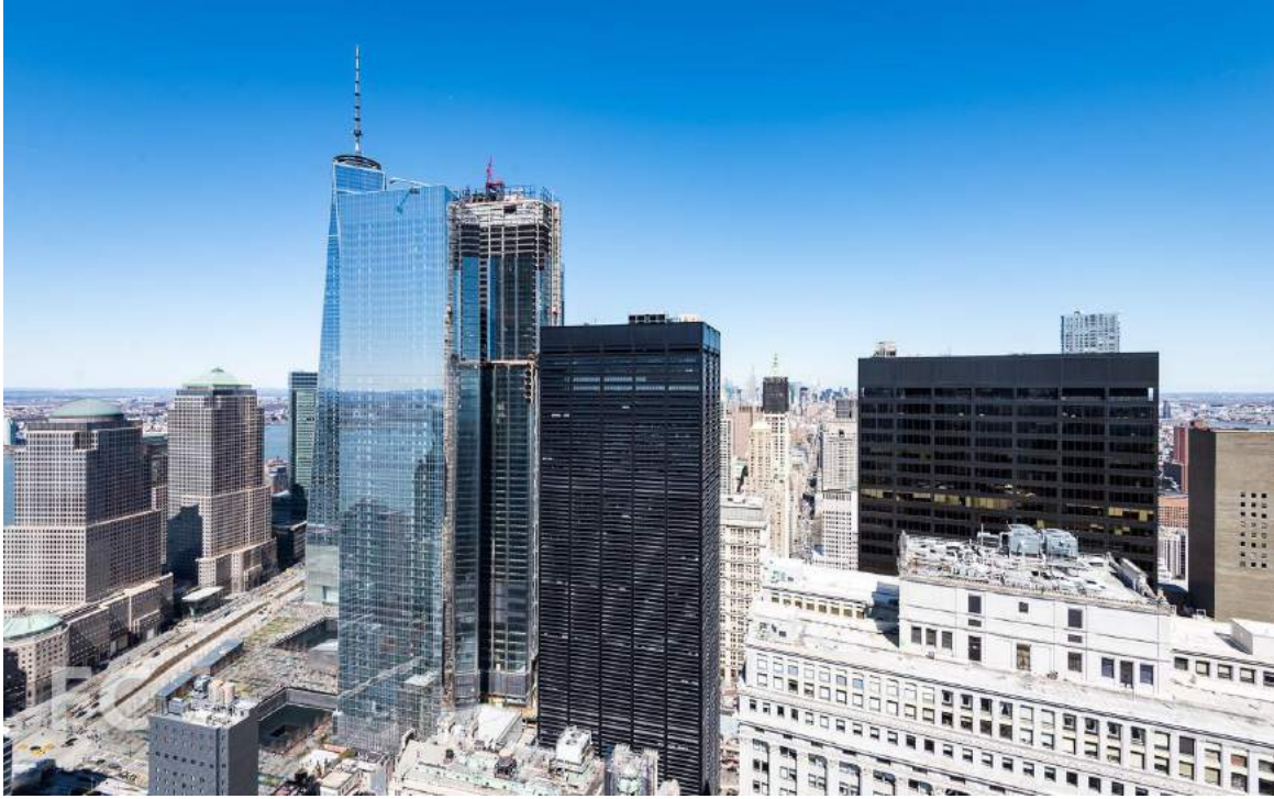
Rooftop view looking northwest.
