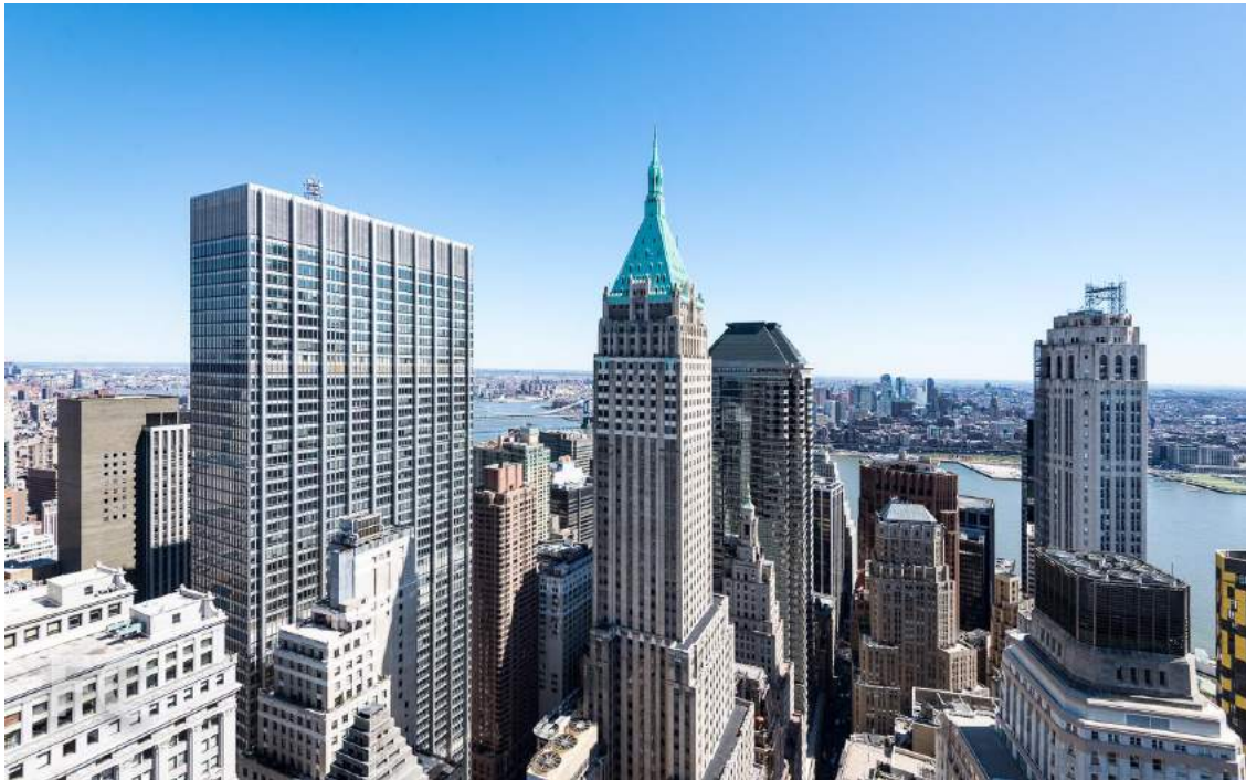
Rooftop view looking southeast.
