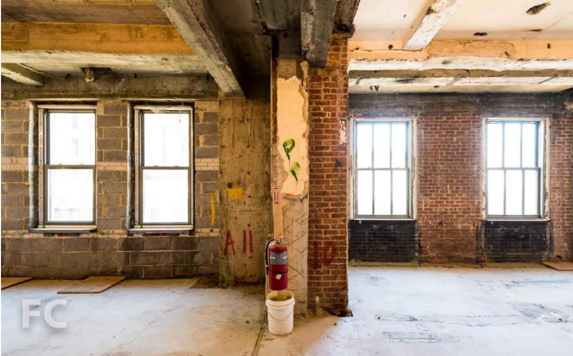
The split between the original 1931 tower (right) and the 1963 addition (left).
