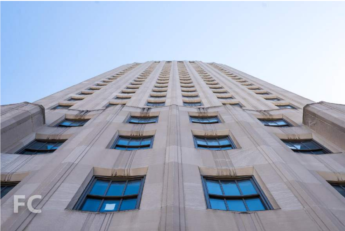
Looking up at the tower from a lower outdoor terrace.
