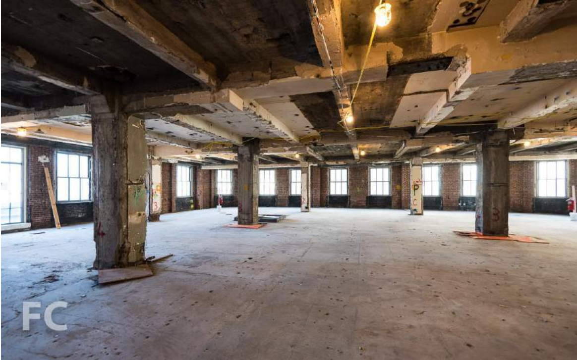
Typical office floor awaits residential conversion.
