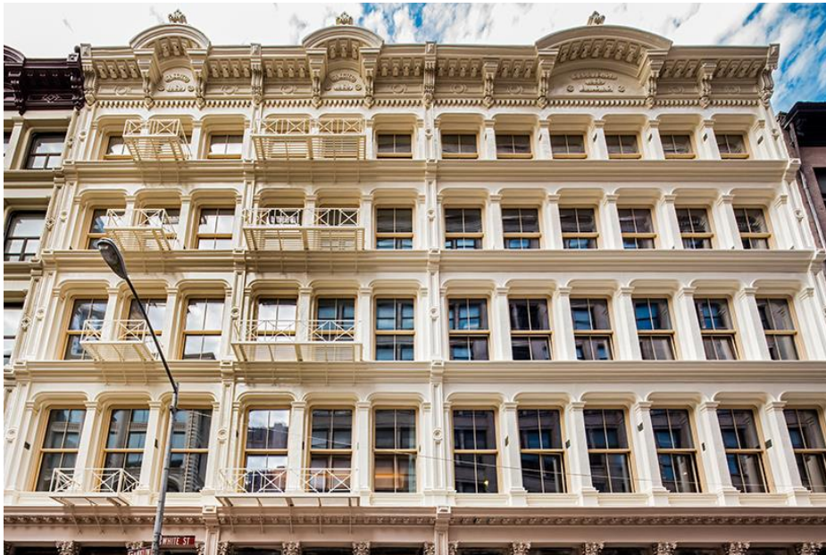
60 white building façade all images © nico arellano
