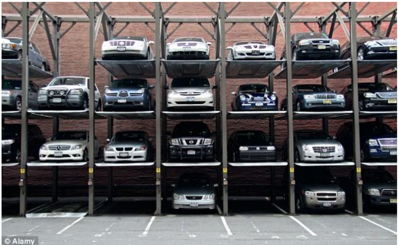
Parking spaces have become so scarce in big cities that wealthy buyers of luxury condos will have to fork out $1million to secure a single spot. Pictured: a stacked parking system in Soho, New York
