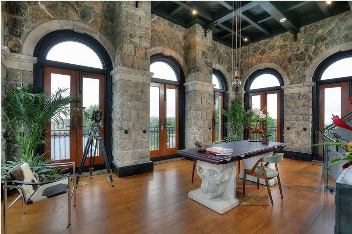
Beyond the stone façade, the interiors were constructed from fieldstone, wood, and terra-cotta, as seen in the study.
