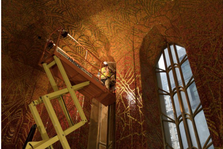
The Red Room restoration in progress. Photo: DBOX for Macklowe Properties
