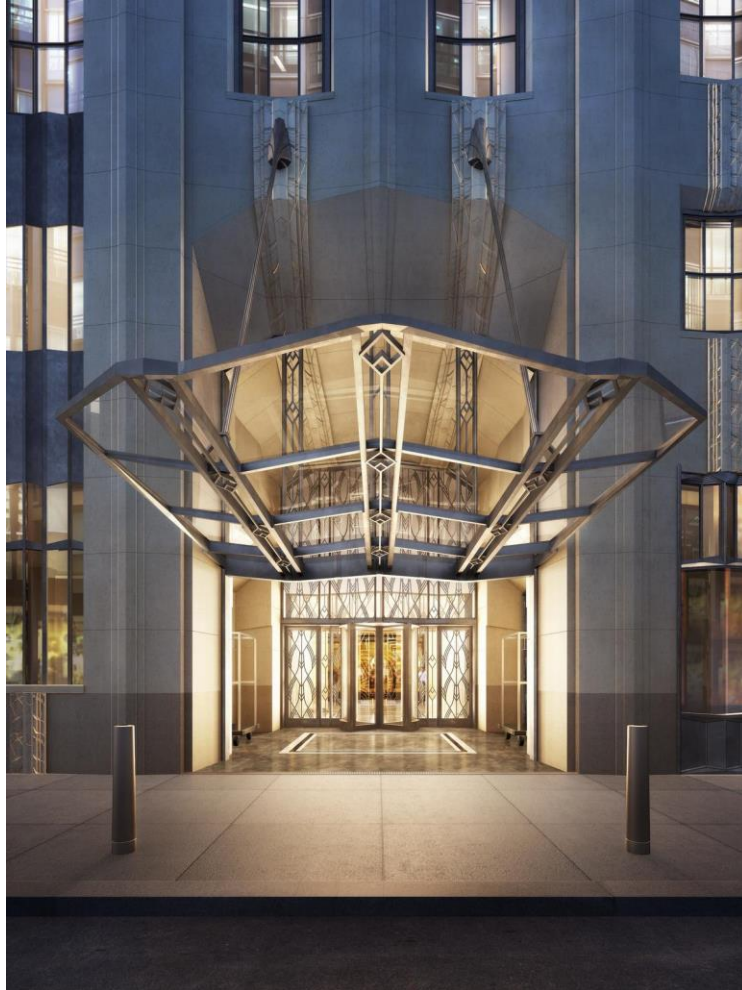
The iconic building was designed in 1931 by Ralph Walker. / Courtesy of Macklowe Properties/SLCE Architects
