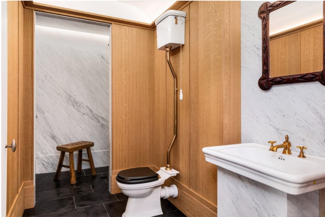
The renovation added a second bedroom and bathroom for Mr. Wendle's sons. The new bathroom features rustic stone flooring and hand-scraped oak wood panels for warmth. TIM WALTMAN/EVAN JOSEPH IMAGES
