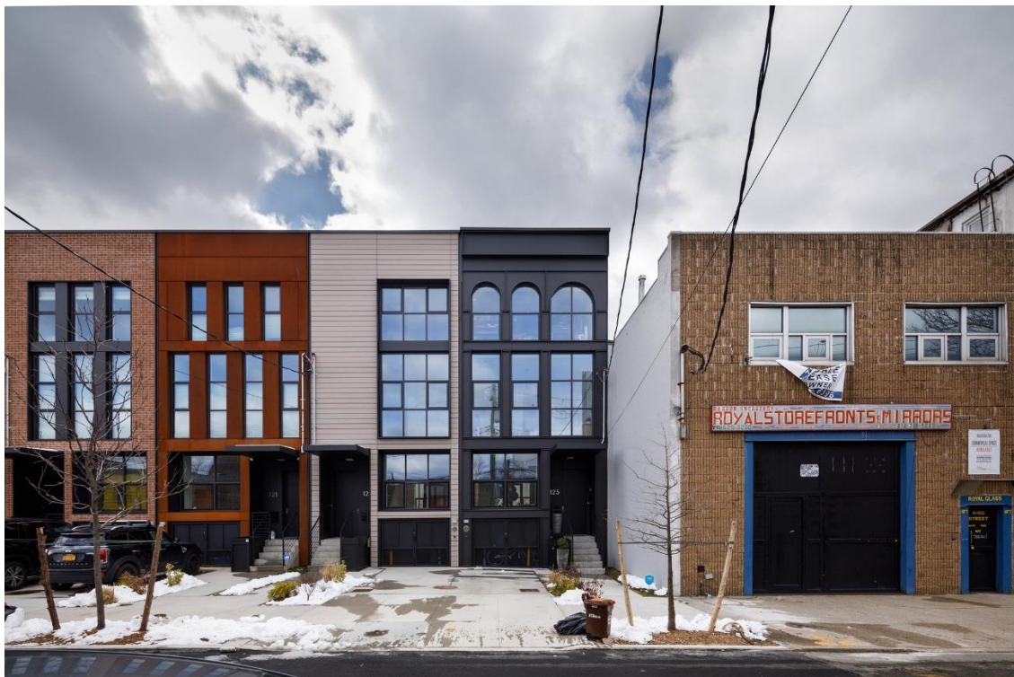
The King and Sullivan development, a 22-townhouse complex, in Red Hook. Stefano Ukmar for The New York Times
