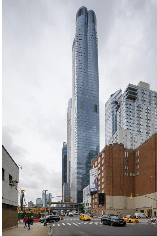
The tower at 15 Hudson Yards, where 37.5 percent of condos had been sold by late August. Credit Stefano Ukmar for The New York Times
