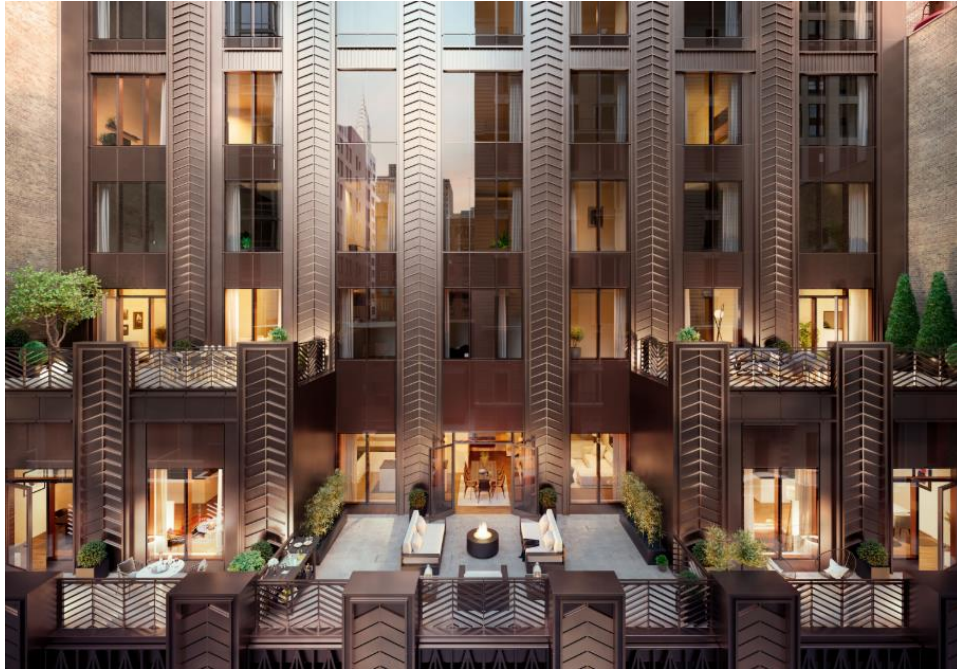
Rose Hill, Art Deco bronze facade, image via The Rockefeller Group and CetraRuddy Architecture
