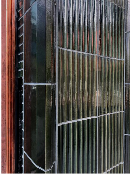
A close-up of the terracotta panels. Photo by Michael Young
