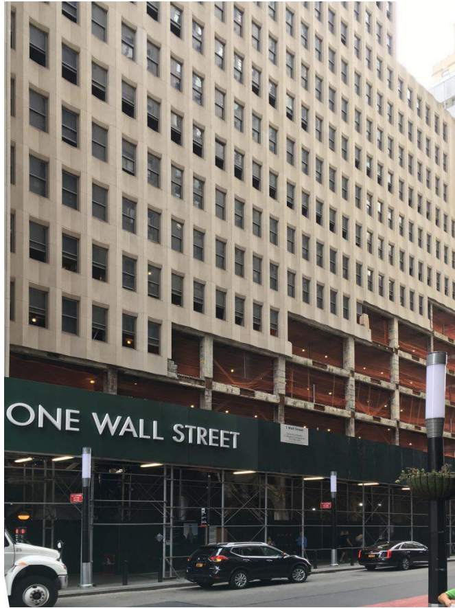
The facade of One Wall Street partially removed at and above street level to make way for the Whole Foods set to come. Photo by Michael Young
