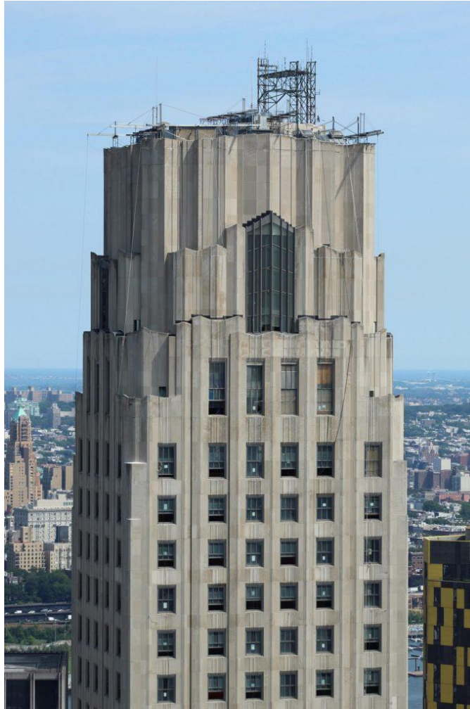
The top of One Wall Street where the triplex penthouse will be located. Photo by Michael Young
