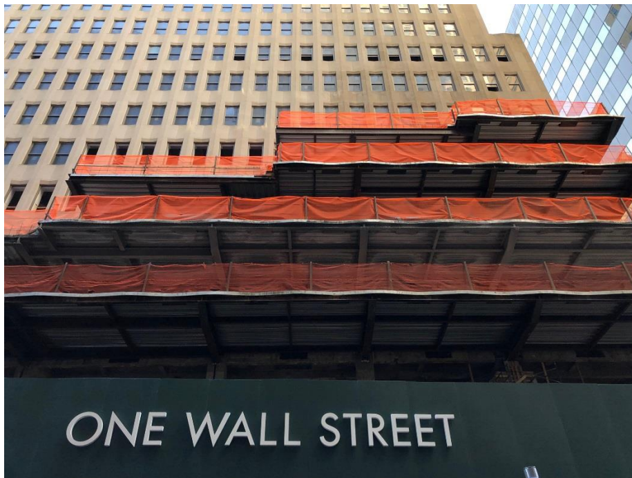
The new retail addition. Photo by Michael Young
