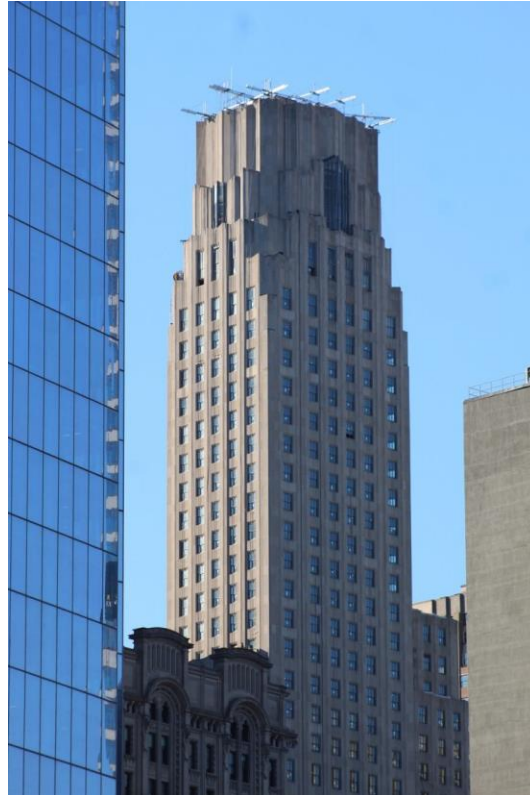
One Wall Street seen from the World Trade Center. Photo by Michael Young
