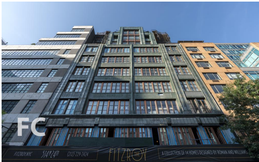
Looking up at the north facade.
