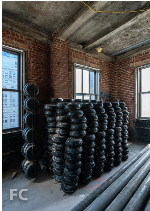
The void elements used in the cobiax slabs.
