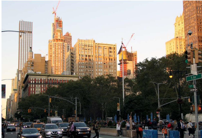
Rose Hill and Madison House condos seen under construction from Madison Square (CityRealty)
