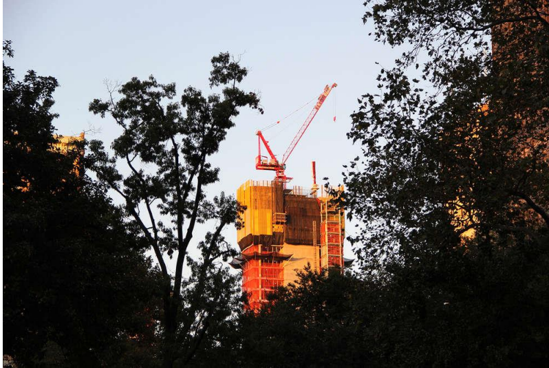
Rose Hill construction beginning to emerge above Madison Square Park (Ondel/CityRealty)
