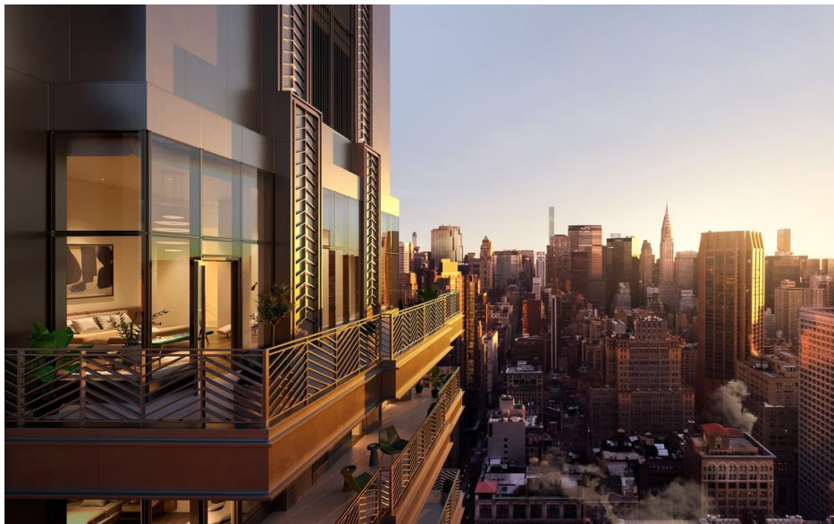
The façade will be clad in bronze-hued aluminium. Image by Pandiscio Green/ Recent Spaces
