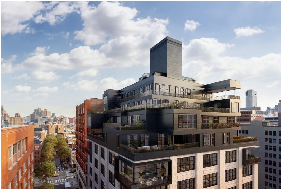
90 Morton is a conversion project in the West Village that added four new floors of cantilevered terraces. Binyan by IF STUDIO
