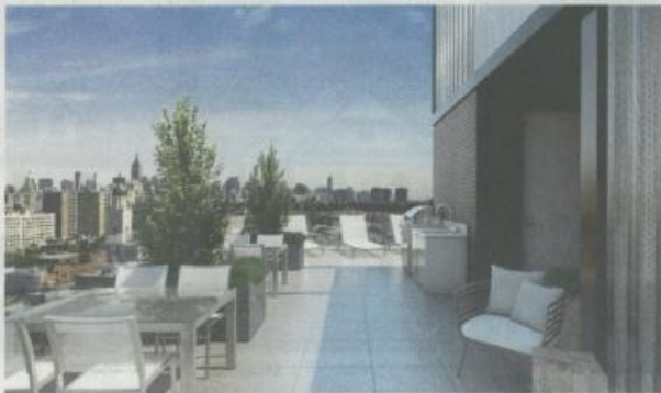
The 11-story, brick-and-steel 287 East Houston Street is rising from a site near Clinton Street. The condo's 28 units will have tall windows and high-end details like Miele appliances. Two maisonettes are planned, each with private outdoor space.
